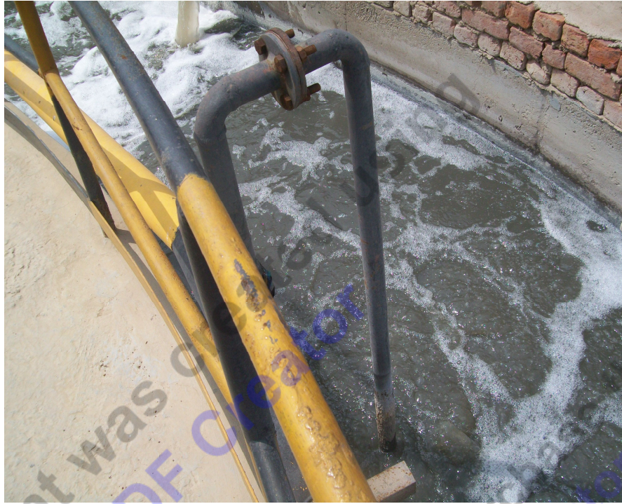
Figure 4.9: Aeration tank at ETP of United Breweries Limited
