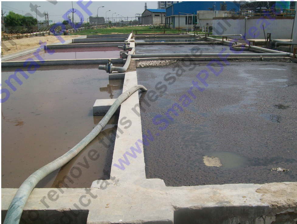
Figure 4.12: Sludge Drying Beds at E.T.P of United Breweries Limited
