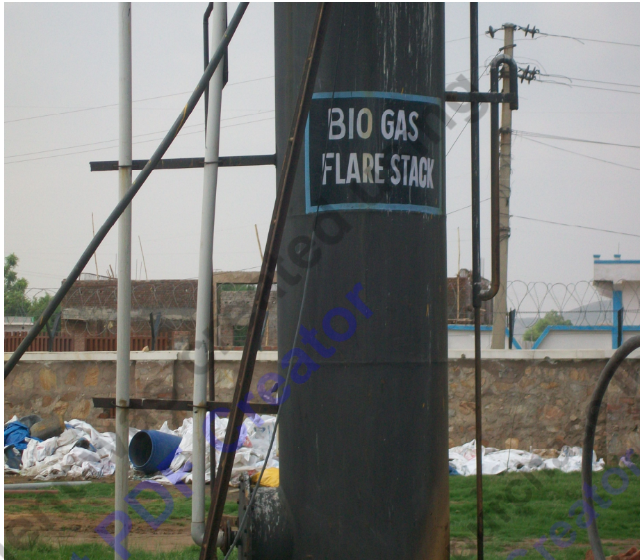
Figure 4.7: Biogas Flare Stack at ETP of United Breweries Limited
