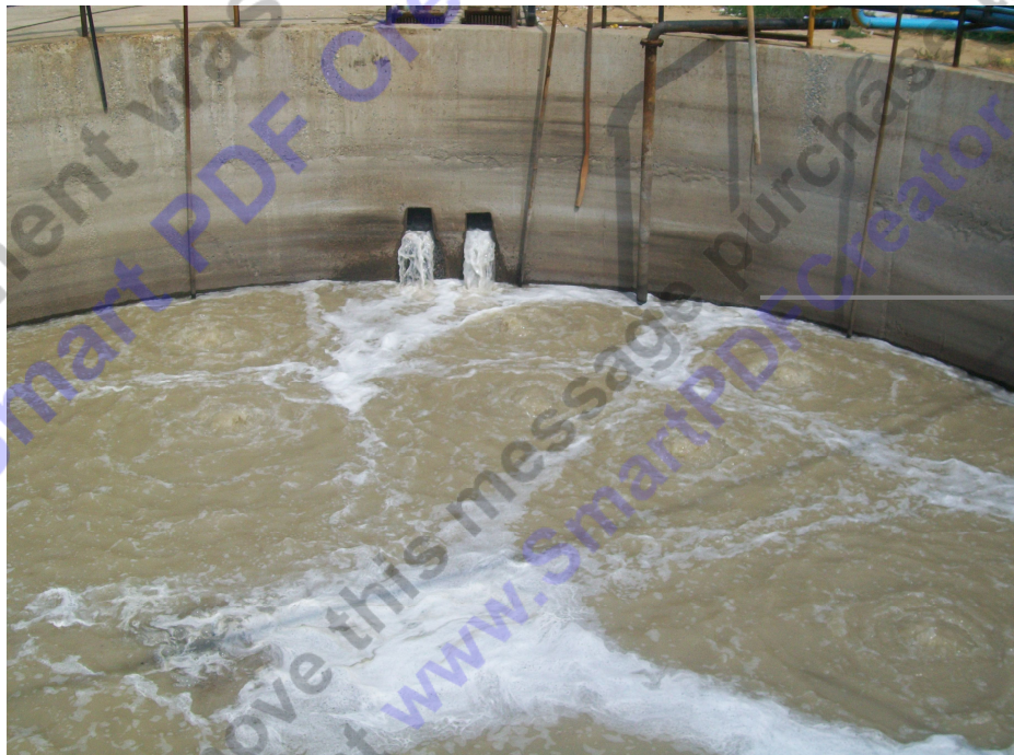
Figure 4.3: Equalization Tank at ETP of United Breweries Limited
