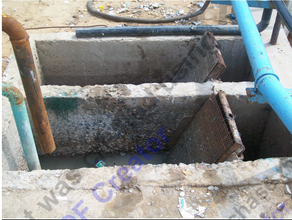
Figure 4.2: Screen Chambers at Effluent Treatment Plant
