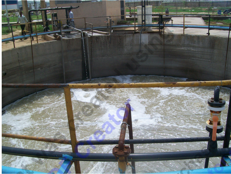
Figure 4.4: Equalization Tank at ETP of United Breweries Limited
