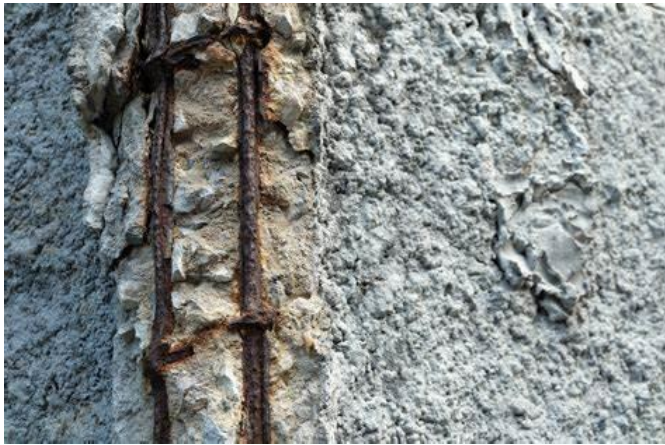
Fig. 4 Chlorides-induced corrosion (Graham 2017)
