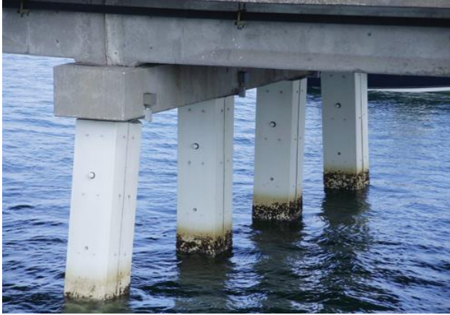
Fig. 3 An RC structure exposed to chlorides (Legault 2011)
