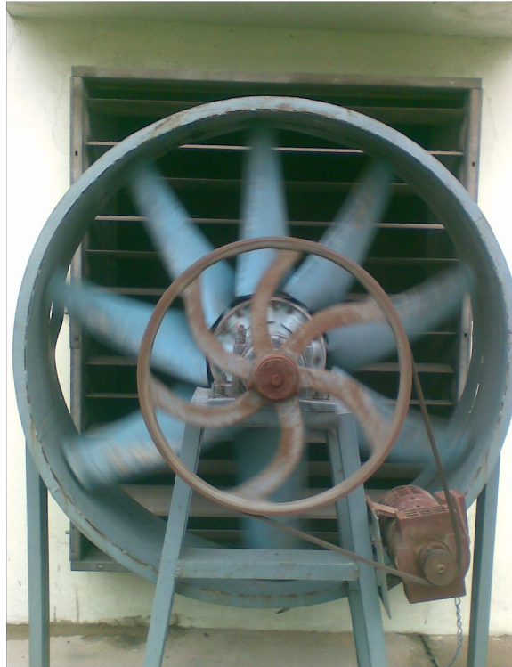
Figure 1. Fan installed in front of the exhaust window. A dynamo can also be seen.
