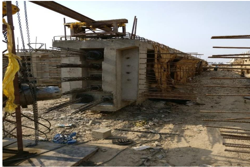
Figure 1. 10 Constructed post-tensioned I girder
