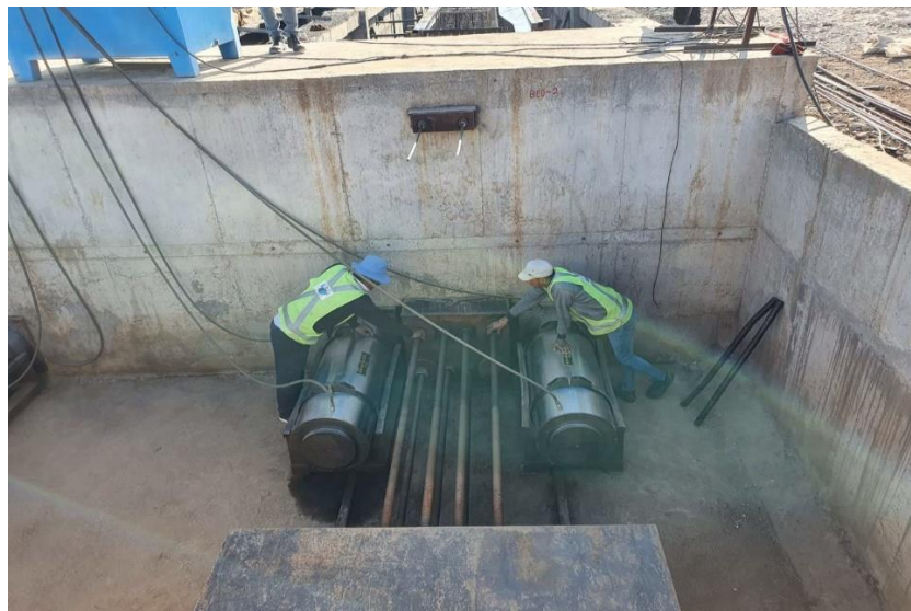
Figure 1. 5 Multi pull jacks and anchor block wall for pretensioned I girder
