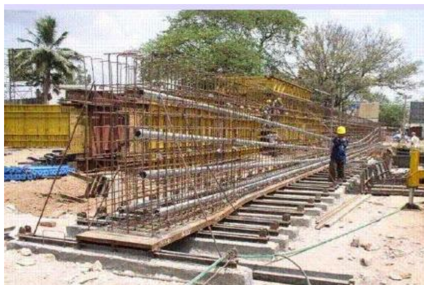
Figure 1. 9 Preparation of reinforcement cage for post-tensioned I girder
