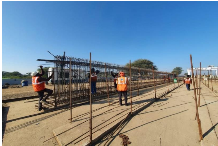
Figure 1. 4 Preparation of reinforcement cage for pretensioned I girder
