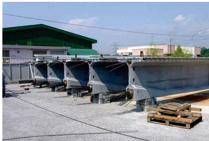
Figure 1. 2 Constructed ultra-high-performance fiber reinforced concrete girder [3]
