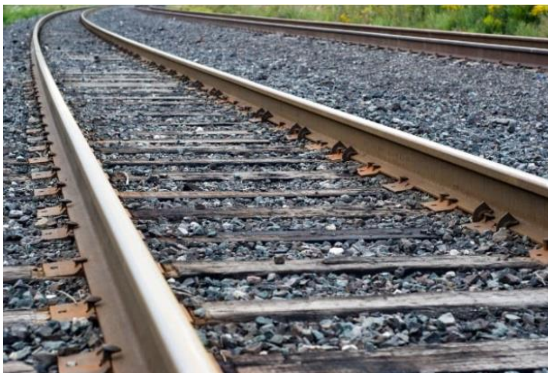
Photo 1.2(b). Continuous welded Rail (CWR)
