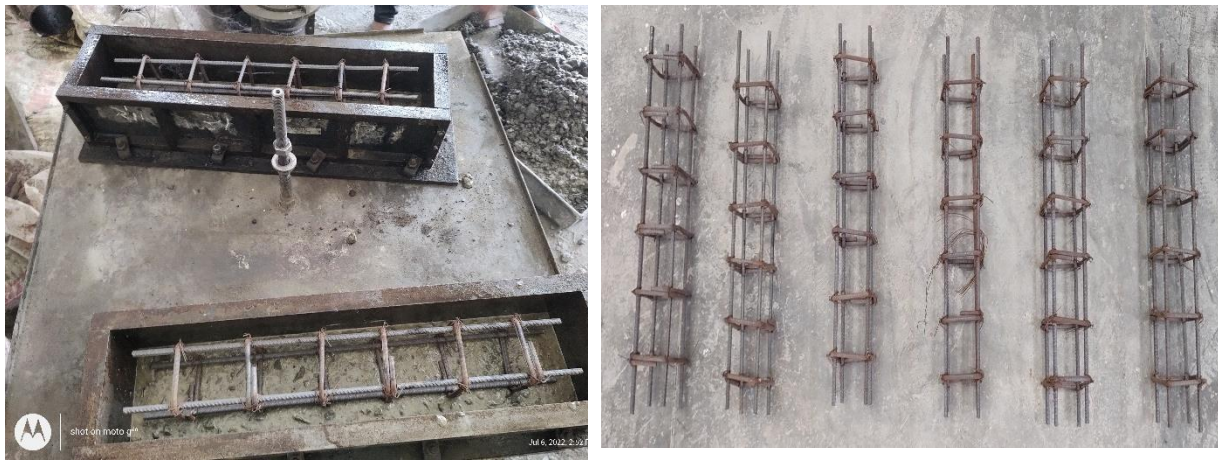
Figure 4. 2 Placing of the JKTPS sensors
