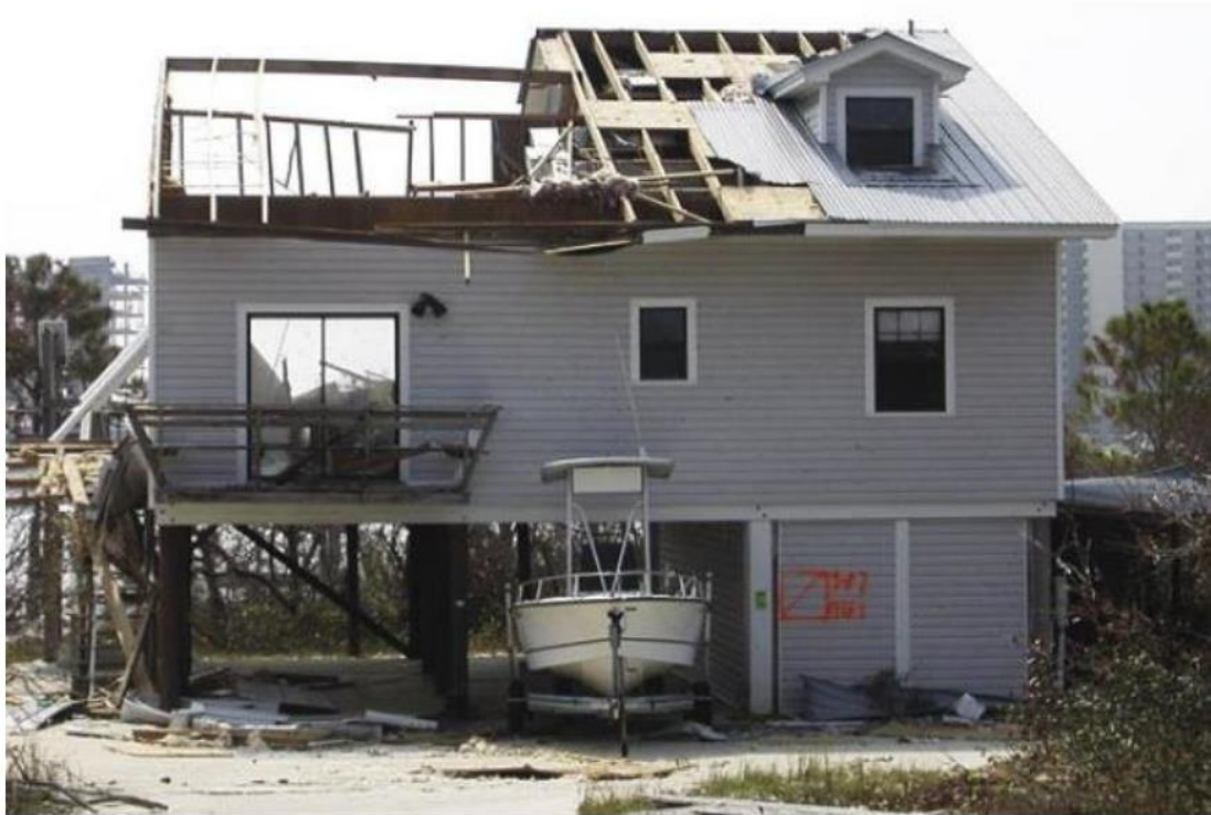
Fig 2 - Structural damage to elevated houses due to the wind during Hurricane Katrina, 2005 (FEMA 549)
