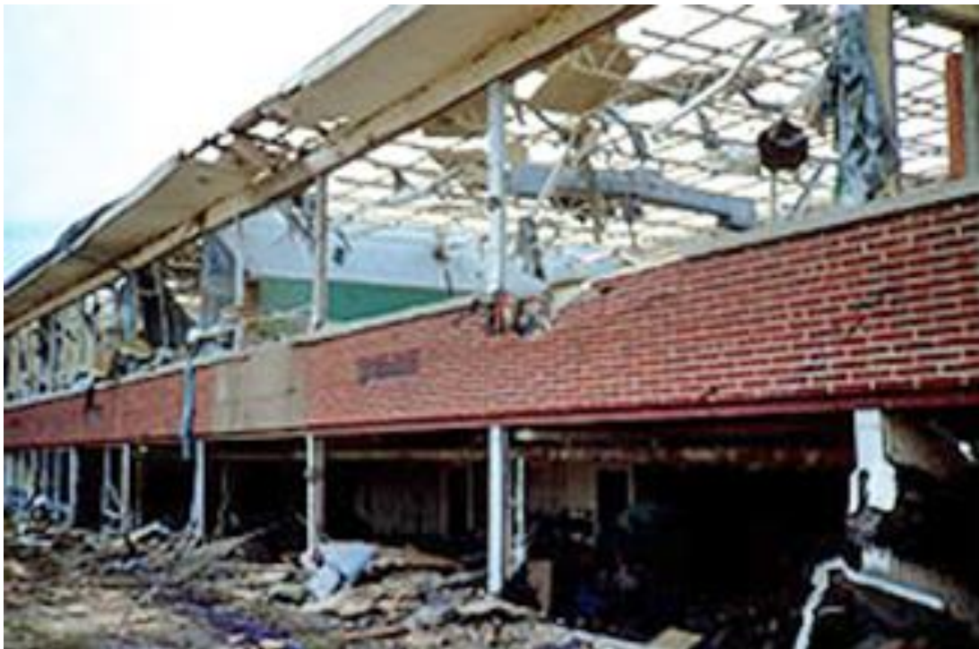
Fig 3 – Damage to building curtain walls during F1/F2 Fort Worth Tornado (2000)
