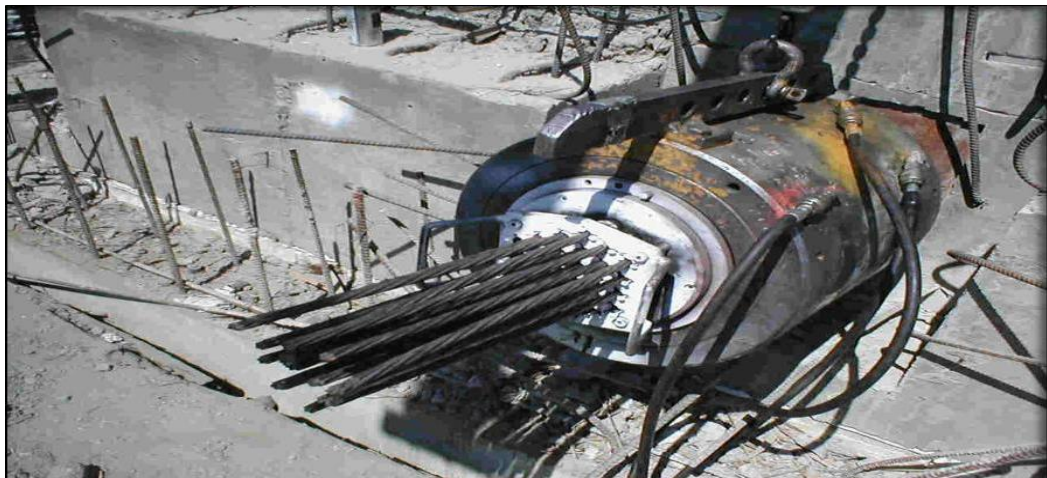
Fig 11: Steel tendons being stretched by jacks in post tensioned members
