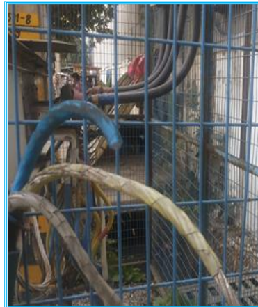
Issues: cracking of R,Y & B ph XLPE insulation & moisture ingress in conventional design
