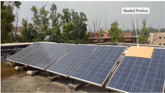
Fig. 10.19: Rooftop PV panels showing partial shading condition.
