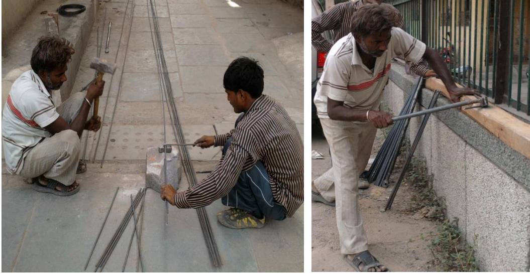
Fig-4.11. Fabrication of reinforcement bars
