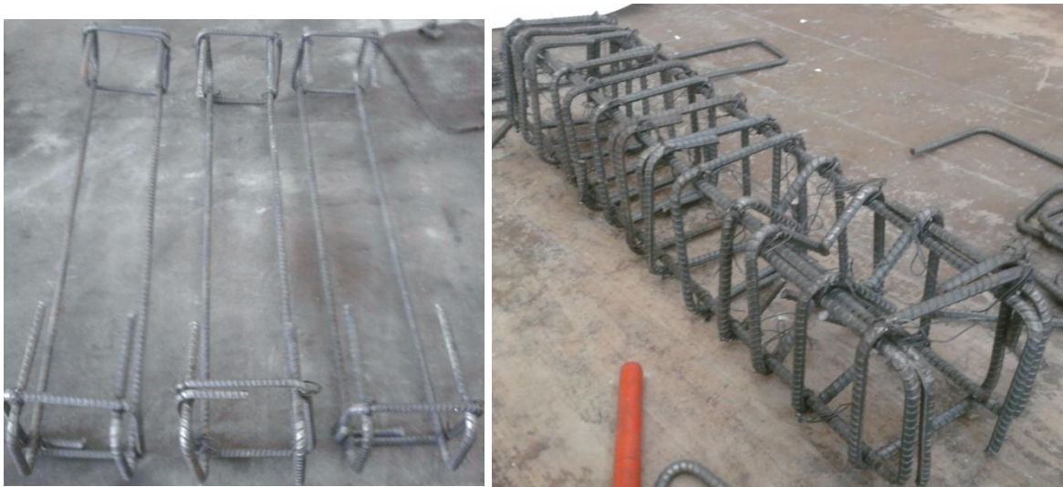
Fig-4.13. Steel reinforcement ready to be placed in beam moulds
