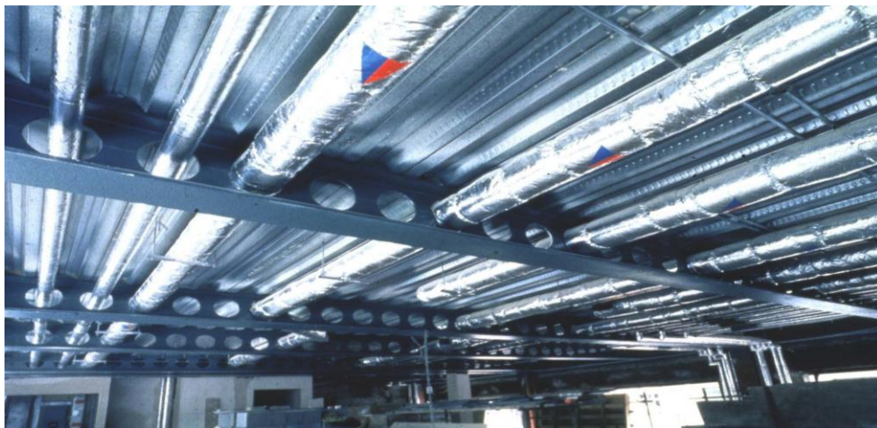
Fig.1.1.Steel beam with transverse opening. [1]
