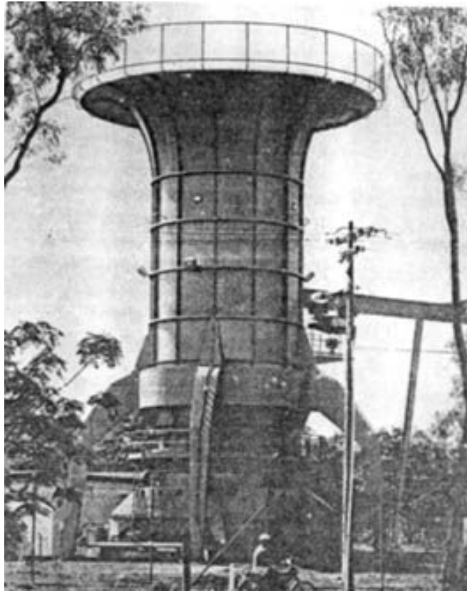
Plate 2. Downcast mine ventilation fan, Mount Isa. (By courtesy of Mount Isa Mines Ltd. Australia.)
